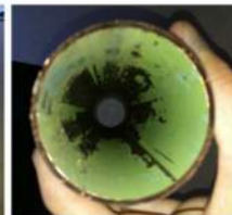
A 2-1/2" diameter hot water pipe was removed from the outlet of the roof-level storage tank. Minor mineral deposits were noted, but generally the sample pipe is in good condition and would not be anticipated to reduce flow. The piping is suitable for substantial continued service life.
